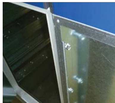
Figure 49: Connection between door frame / internal panel
