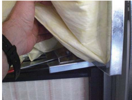
Figure 91: Lifting the filter bags
