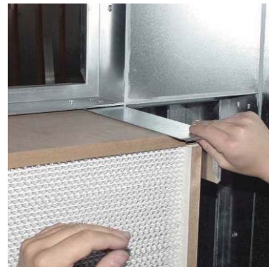
Figure 93: Inserting the filter cell
