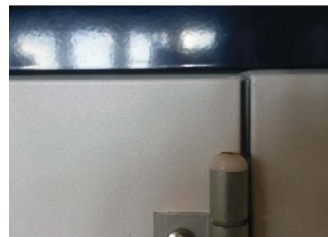
Figure 81: Adjusted – constant slit width
