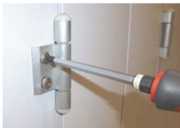
Figure 80: Adjustment of the door panel
