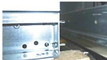
Figure 51: Application of self-tapping screws
