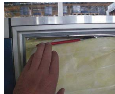
Figure 90: Clamping the filters
