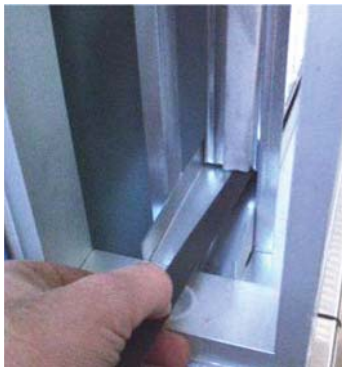
Figure 83: Pulling out the filters
