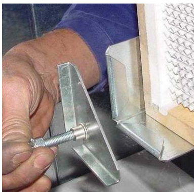
Figure 94: Inserting the clamps
