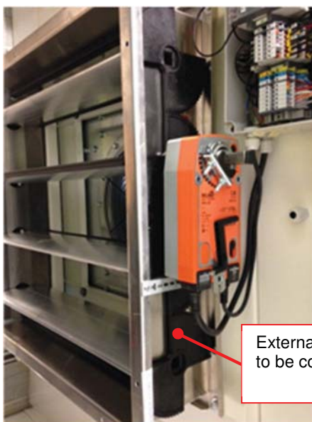
Figure 96: Damper with external gear wheels
