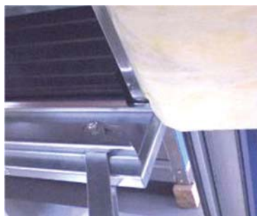
Figure 89: Slide in the filters
