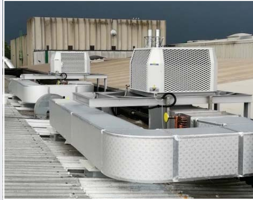
Waste treatment plant, Italy
